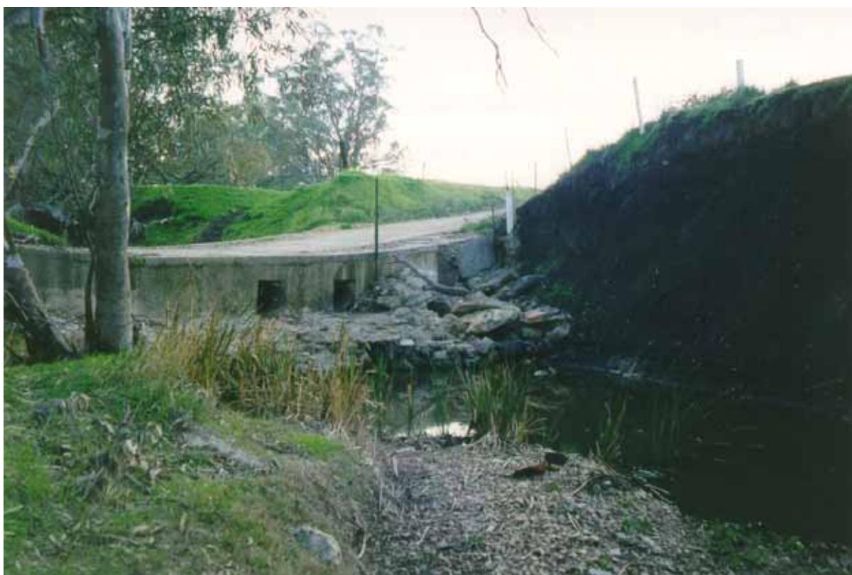
Plate 5.10: Poorly positioned and undercapacity culvert causing bank erosion and scouring downstream, Skillogalee subcatchment.
